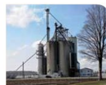
Grain dryer farm operations in the area
